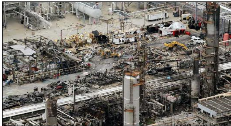
Explosion leading to multiple fatalities and major asset damage
