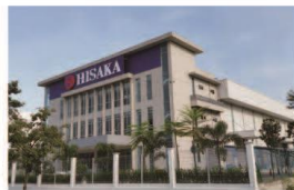
HISAKA WORKS S.E.A. (Malaysia)
