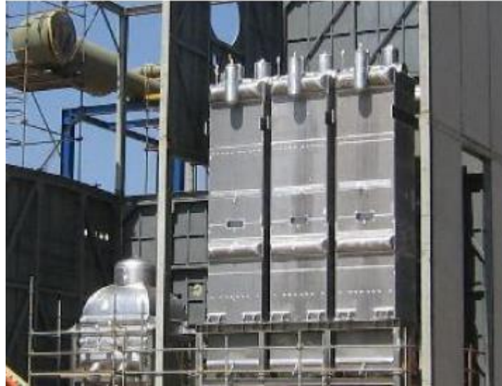
Configuration of Plate heat exchanger
