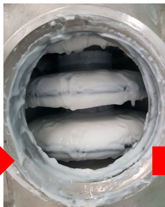
Heat is applied: jacket 90C, hot N2 90C (1 hr during separation and bone dry cake)
