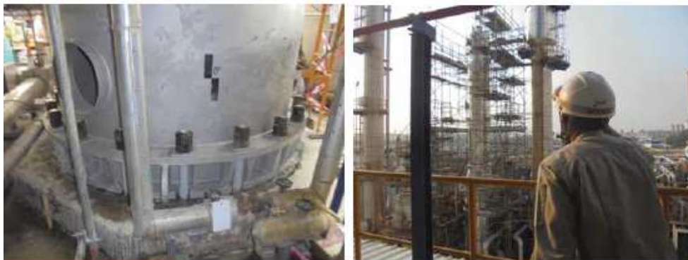
Column vertical alignment inspection
