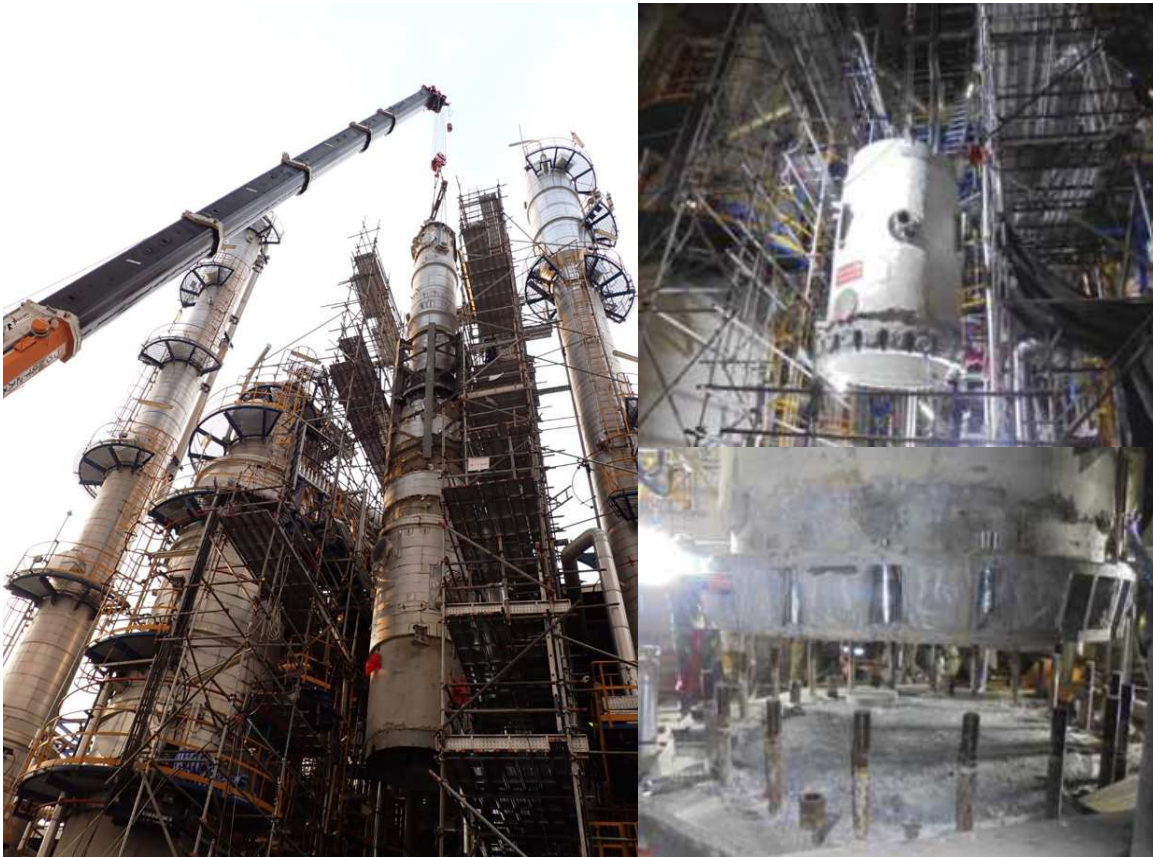
Existing column Removal : Focus to avoid anchor bolt and padding damage
