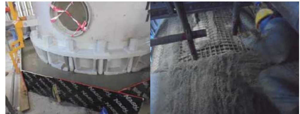
Grouting and Fireproof
