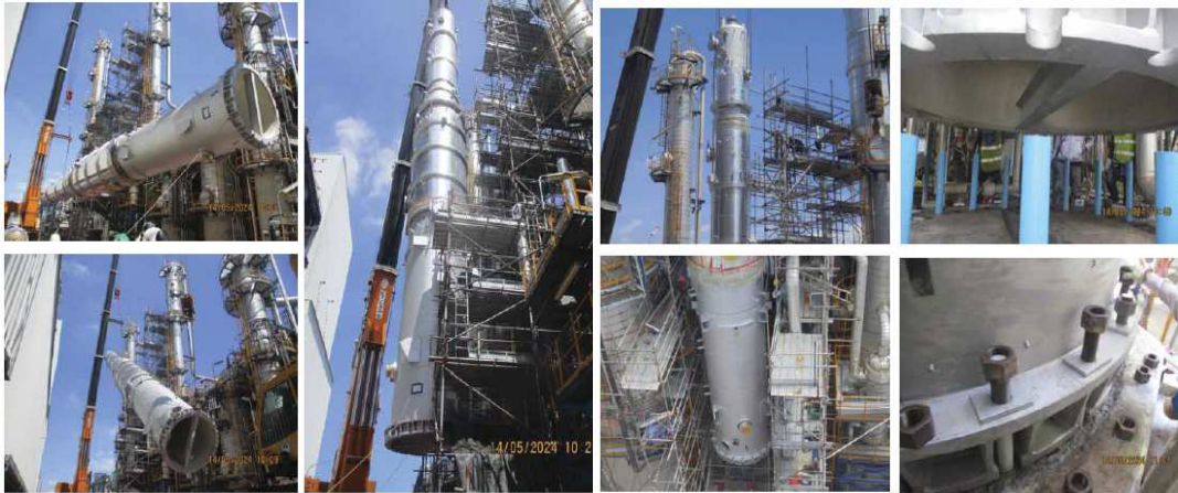
New Column Installation
