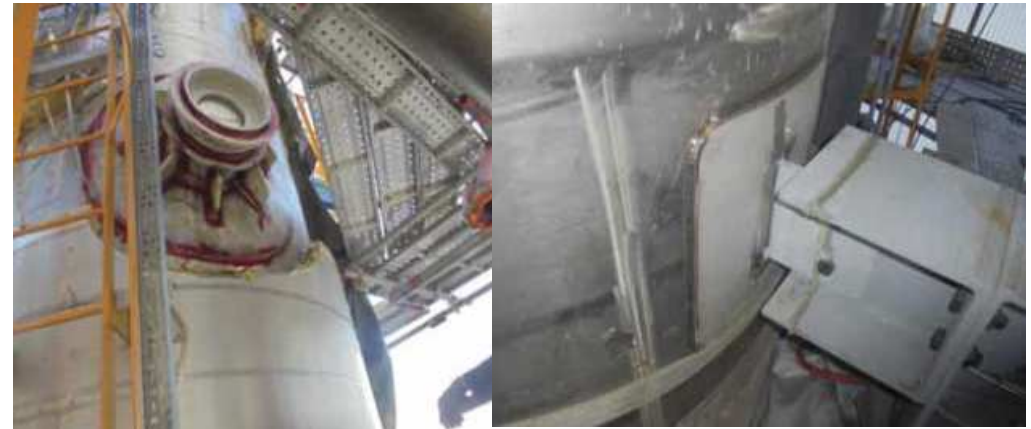
Lifting Preparation : NDE Lifting Eq. and Weld external support
