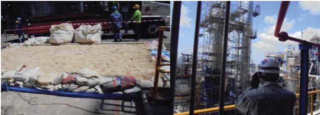
Site Preparation : Rigger plate preparation and plumbness check
