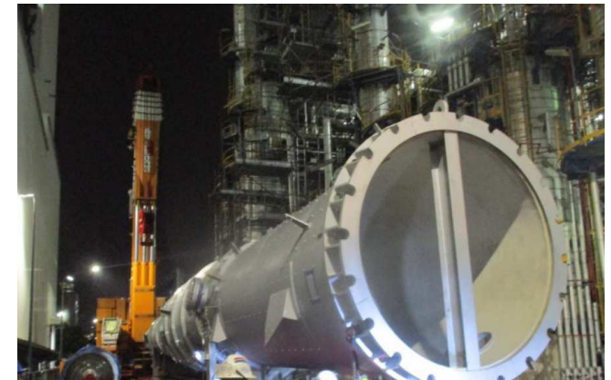
Transportation : New Column Available on Site
