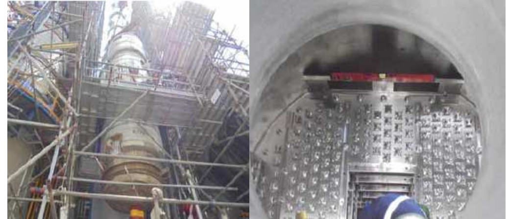
E-1701 Re-Installation and Internal tray final inspection
