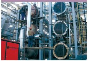
**ESSAR OIL** UK, Diesel Rundown Cooler
