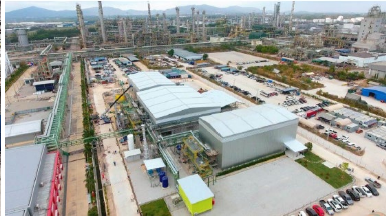
Circular Plas Co., Ltd Demonstration Plant in Rayong
