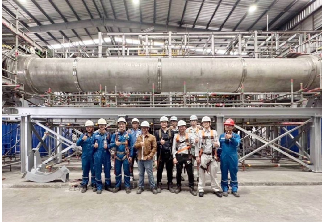
Successful Installed The New Type of The Reactor at Circular Plas Co., Ltd
