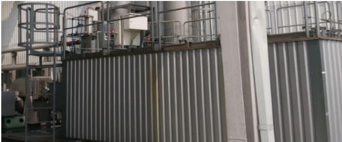
Printing air Air volume: 7,000 Nm 3 /h
