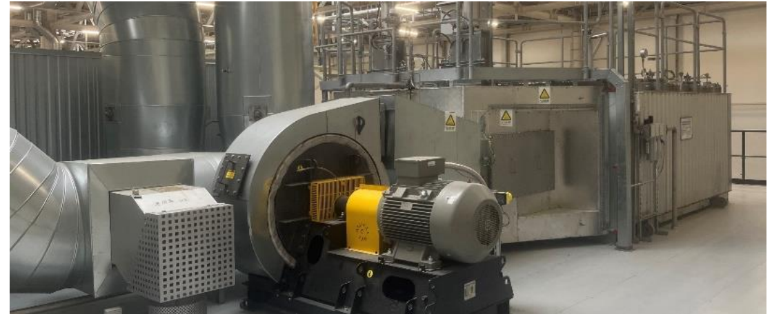
Car body oven Air volume: 1 x 9,000 Nm 3 /h
