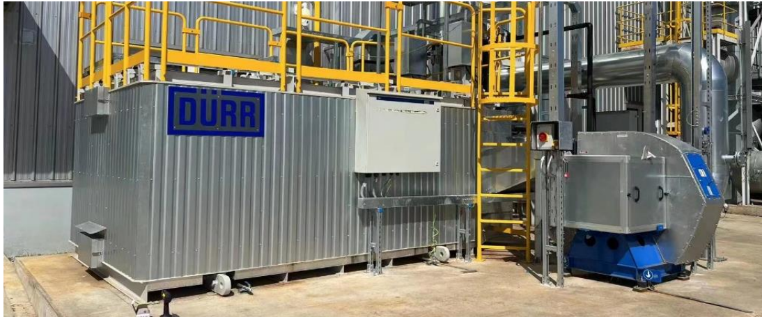
Foam exhaust Air volume: 4,500 Nm 3 /h
