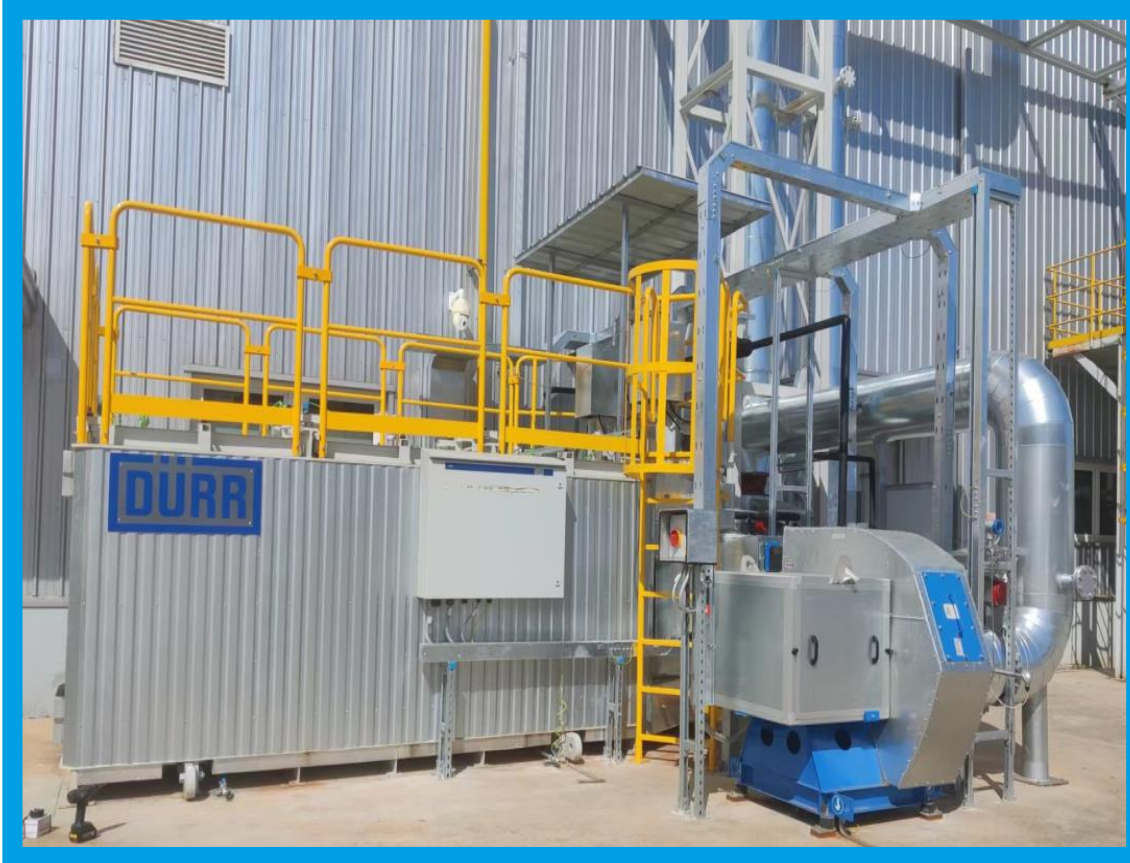
Oxi.X-RV 0813, flow rate 8000m 3 /h
