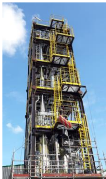
DMX™ demonstration plant Arcelor Mittal, Dunkerque 500 kg/h CO 2 capture
